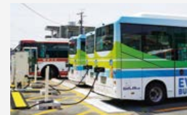
EV Bus Charging Management System
